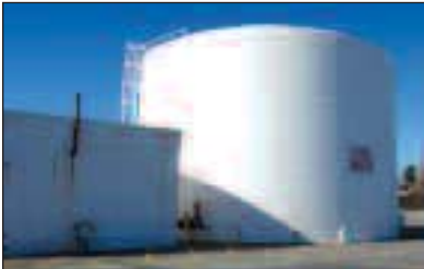
300,000 Gallon Water Storage Tank
